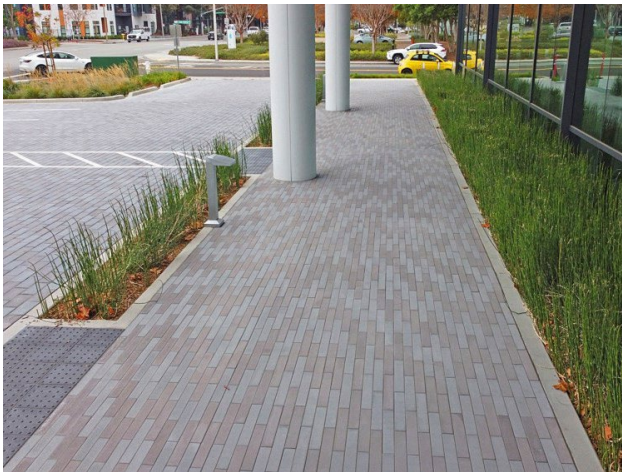
Unit Paver 1, Permeable Narrow Modular Pavers (3" X 9"), Stepstone in medium shade (See below)
